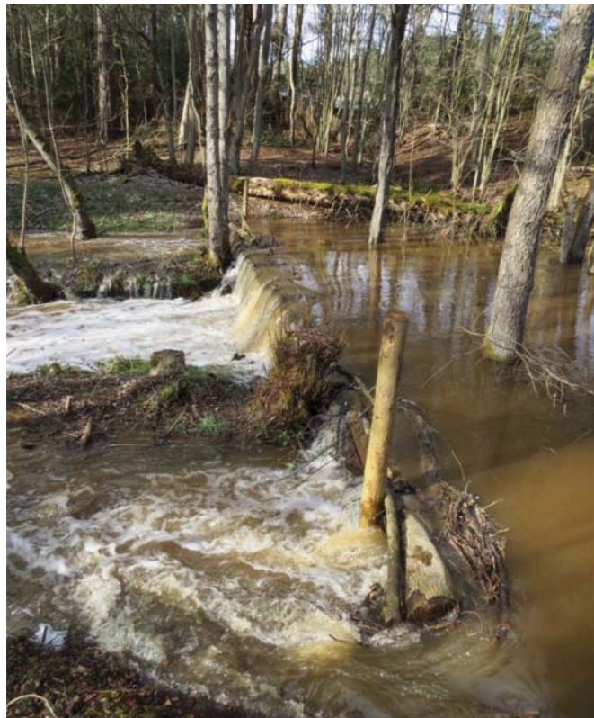
A leaky woody structure holding back flood waters during a flood event on the Pickering Beck in North Yorkshire. (Photo: Tom Nisbet)
